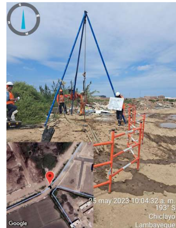
Sondeo SPT: "Wash-Boring"
